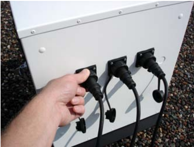
Figure 42: Connect Power from the Solar Cell Power System to the Environmental Enclosure
