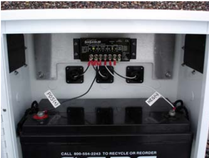
Figure 33: Install the Solar Battery and Connect to Controller
