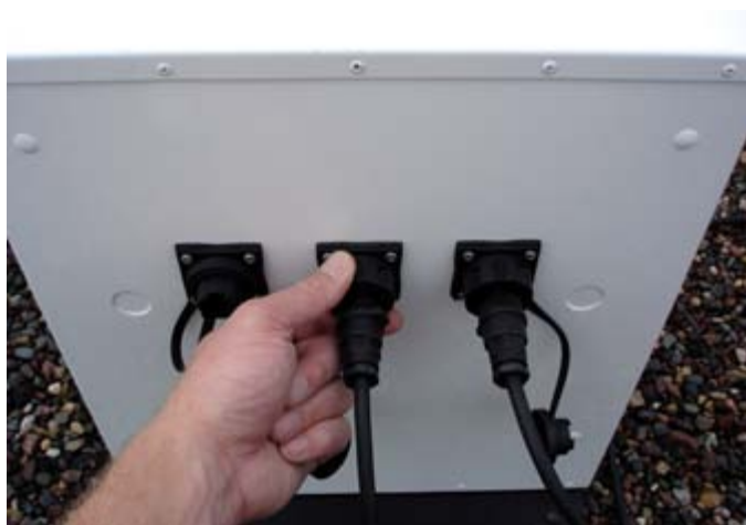
Figure 41: Connect Solar Cells to Battery Enclosure Box
